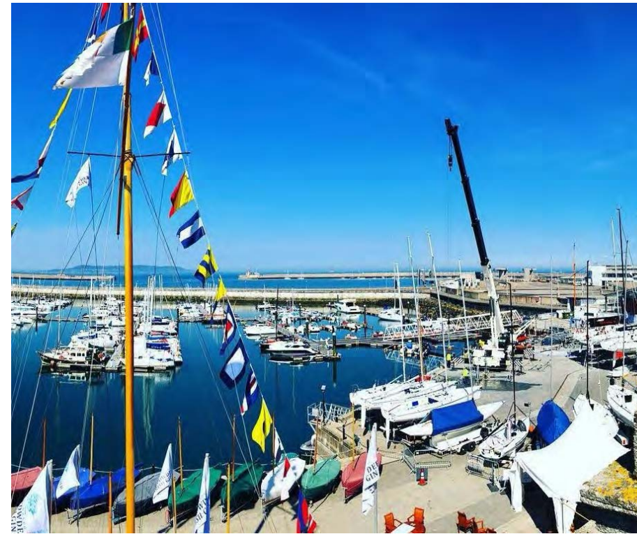
Liebherr 90 tonne crane
